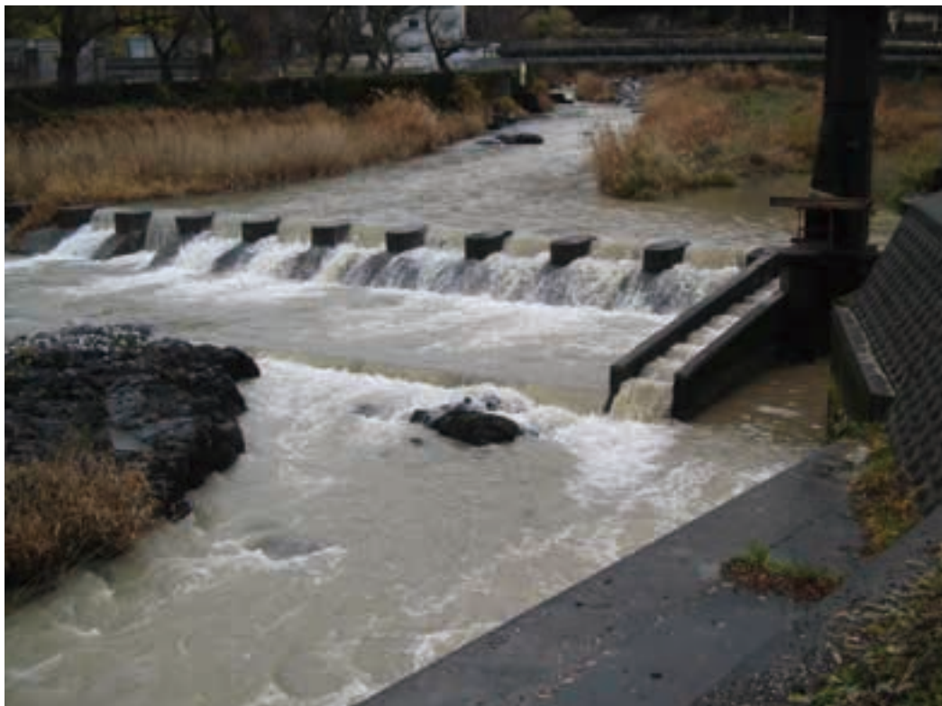
頭首工と魚道 Headworks and fishway
